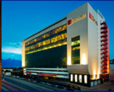
Monterrey, MX November 7-9
